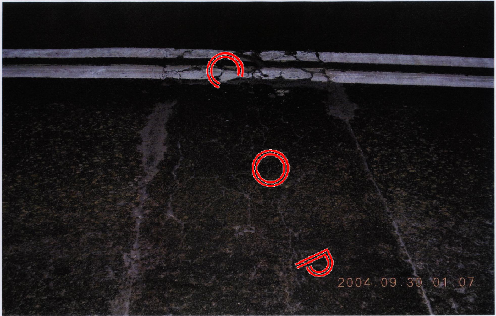
Figure 4 - Damaged Asphalt at Cross Drain
