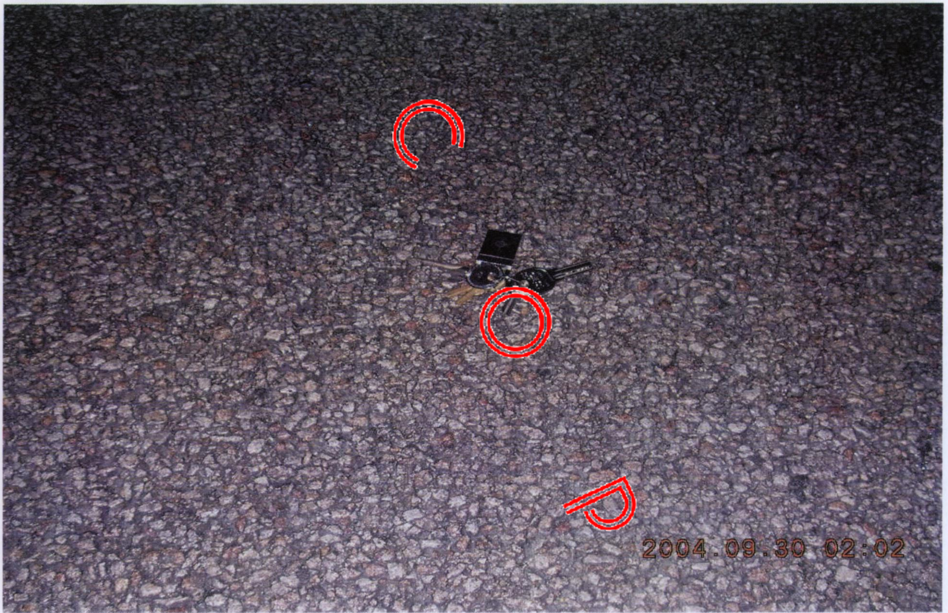
Figure 5 - Exposed Pebbles in Asphalt Pavement
